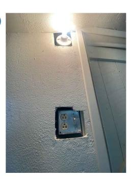
15.4.1 Ceiling, Walls & Firewalls in Garage **POOR PATCHING OBSERVED** Recommendation **Contact a qualified professional.**
